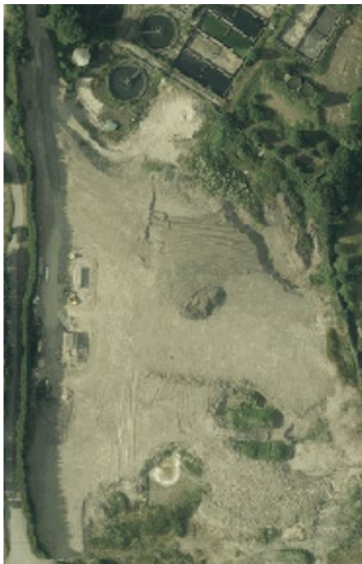
Figure 3 - aerial imagery from 2018 after the water works had been removed.
