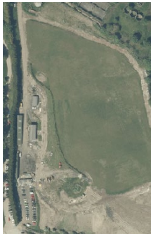
Figure 4 - aerial imagery from 2021. The proposed building can be seen in situ to the west (left).
